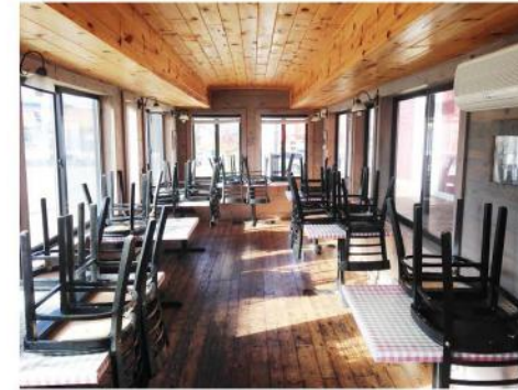
Left: The space was formerly Lester’s BBQ. Right: The floor needed to be leveled with concrete and a reclaimed hit-skip pine was added.
